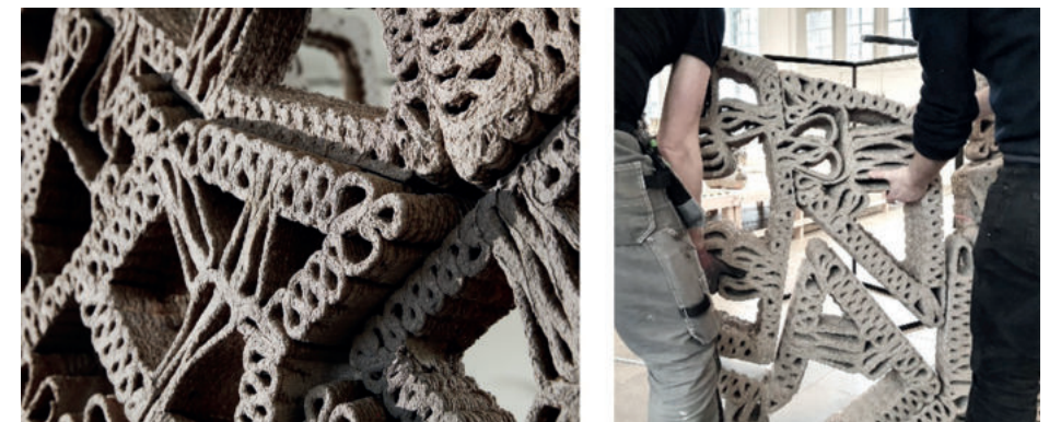
Fig. 3: Close-up details of Cellulose Enclosures. The interlocking of the structure is guaranteed thanks to the male-female joinery as well as the component outlines which stack in compression.
