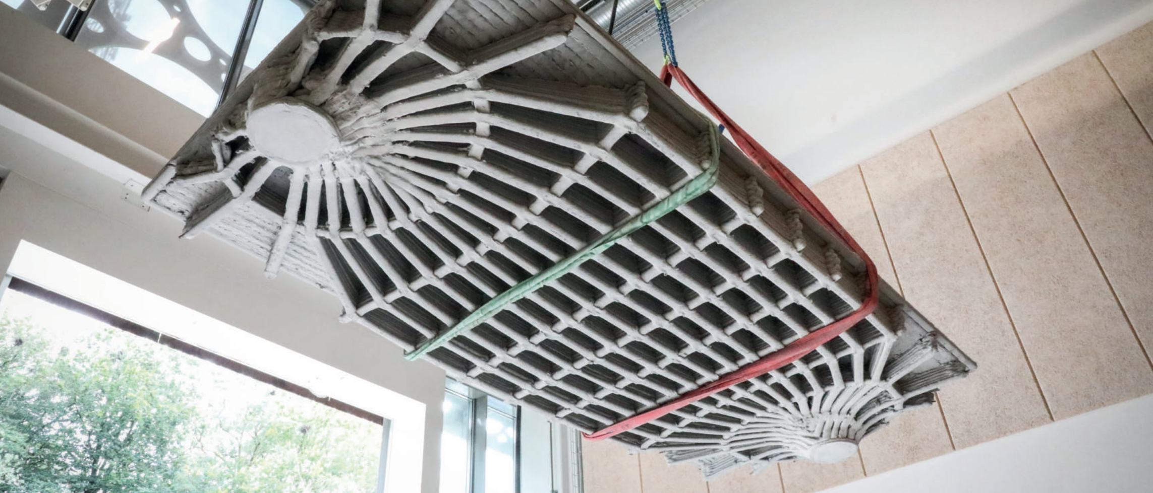
Fig. 6. Outlook of 3DLightSlab, a 3.5 m x 1.6 m ribbed slab with two punctual supports and optimised through PML and non-planar 3DCP extrusion
