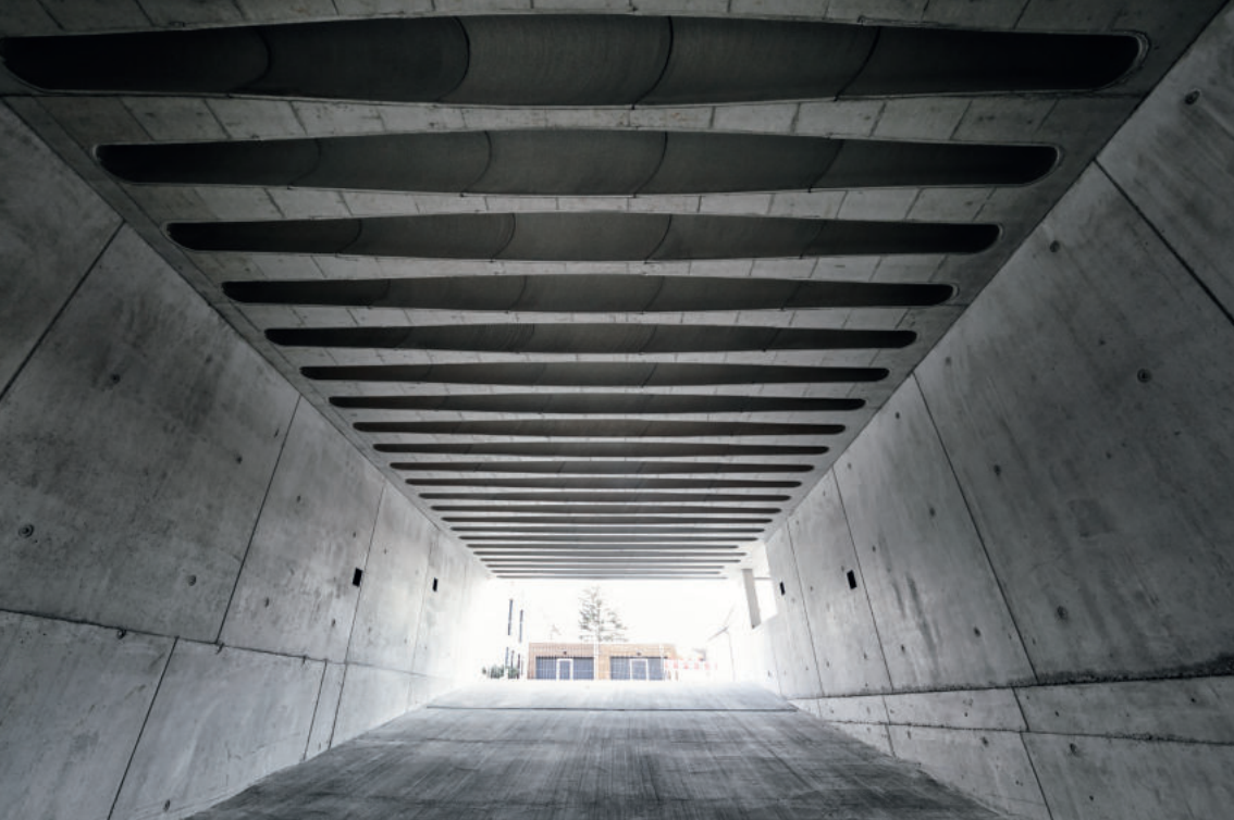
Figure 6: roof construction-inside view
