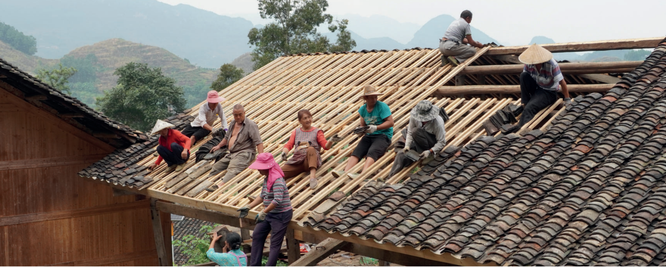
Fig. 9: Reintroduction of wooden structure and roof
