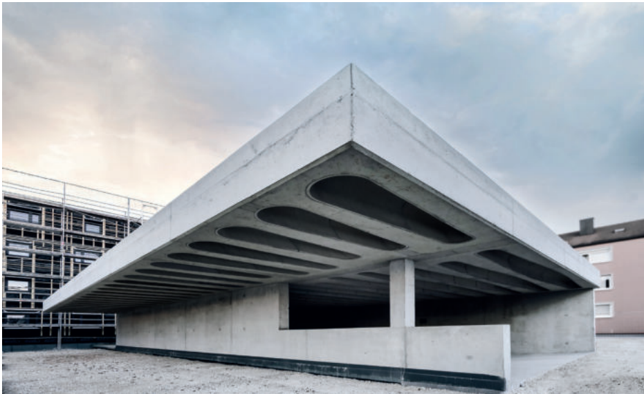
Figure 2: Realized building project in Nördlingen with a 170m 2 material reduced slab
