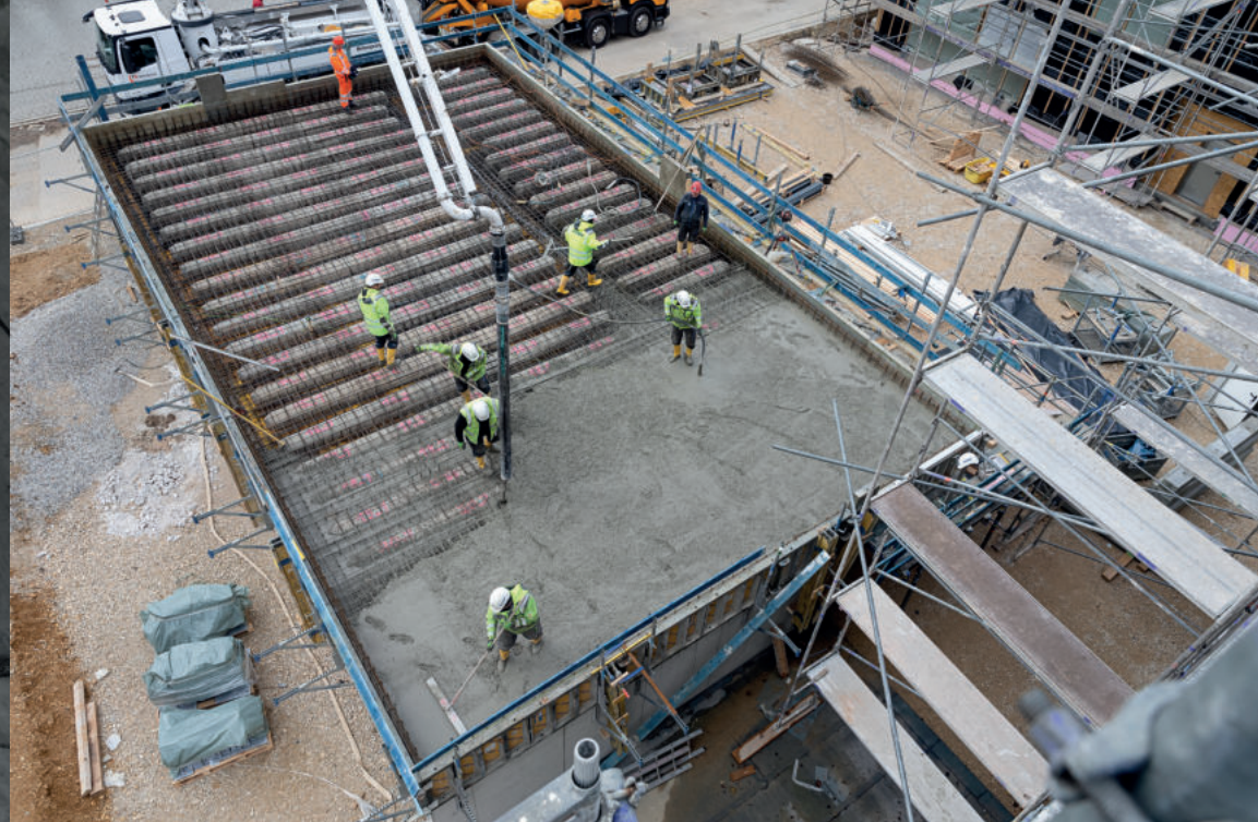
Figure 7: roof construction- building site
