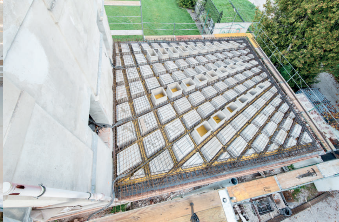
Figure 5: 3D printed void bodies placed on the formwork table
